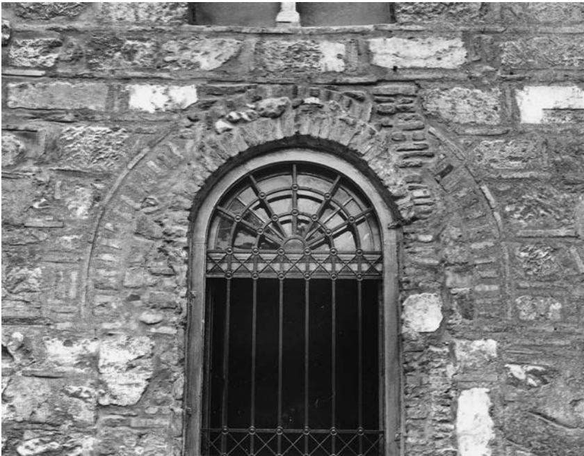
Figure 212 Katholikon of the Petraki monastery. The north main door. The three different phases are obvious.
